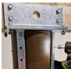
Skruva fast toppbeslaget till stolpen Screw the top bracket onto the post
